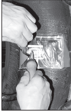
10. Stitch the repair onto the prepared area. Stitch from the center of the repair to the the outside to remove any trapped air.
